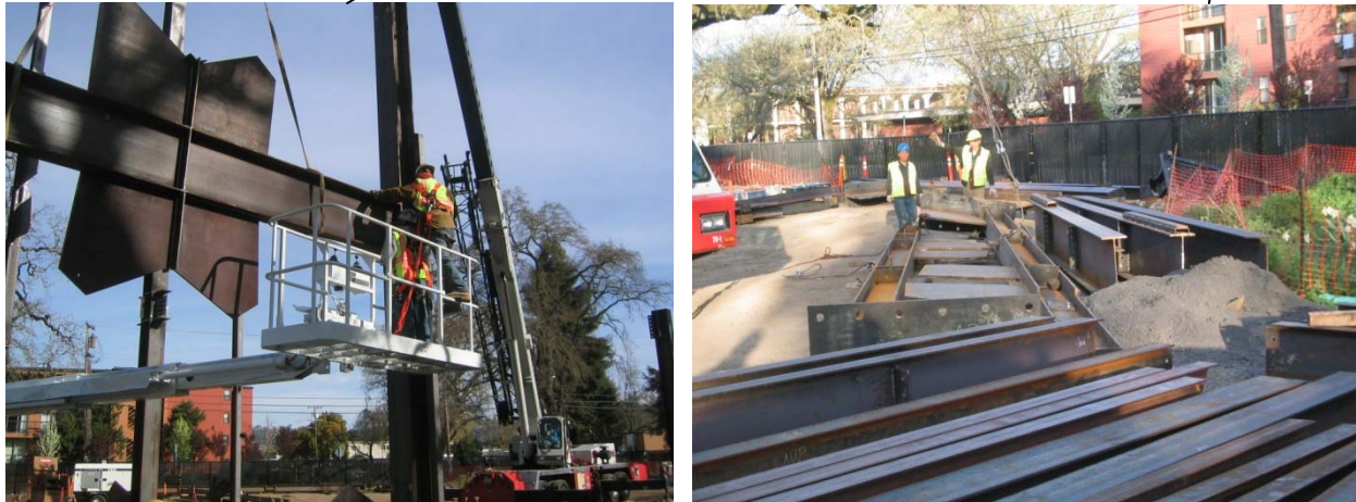
Above: Steel being set by crane in section 1
