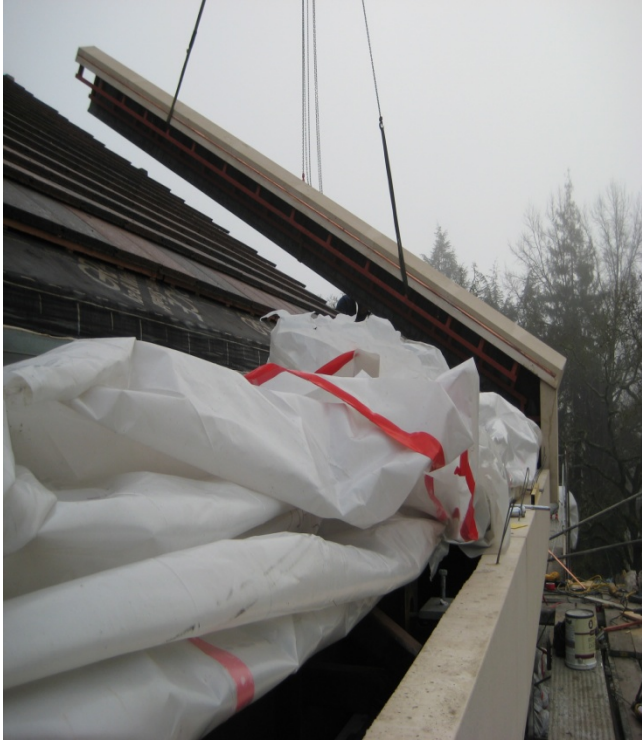
Above: Precast concrete panel being lowered into position
