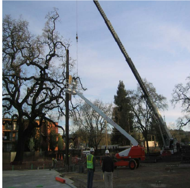
Above: Single crane and crew used during erection process
